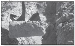
Bury the Savio Aqua Flex PVC<sup>™</sup> below freezing level by digging a trench (shovel width) 10" below existing ground level along the pond perimeter from the Savio Skimmerfilter<sup>™</sup> to the Livingponds Waterfall Filter<sup>™</sup> or water return.
