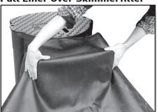
Position pond liner over the Skimmerfilter $^{\text{TM}}$  mouth and hold it in place. Smooth liner free of wrinkles and folds. Wipe clean.
