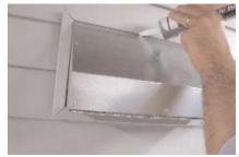
APPLY A BEAD OF CAULK AROUND HOOD AND SIDING.
