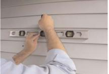
DRILL (4) 1/2" CORNER HOLES THROUGH WALL FROM INTERIOR AND CONNECT HOLES ON EXTERIOR WITH A LEVEL. ALIGN TEMPLATE WITH HOLES AND TRACE REMAINING LINES.
