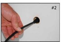
using an extension cord, it must be a 3 wire, 18 gauge (outdoor rated) grounded plug cord. Be sure the connection is elevated off any surface and not near water.
