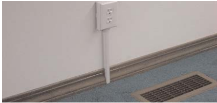
FINAL SURFACE WIRING INSTALLATION WITH ASLL.
