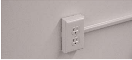
SURFACE WIRING CAN ALSO BE RAN HORIZON- TAL IF THERE IS NO ELECTRICAL OUTLET IN THE JOIST/TRUSS CAVITY ASLL WILL BE INSTALLED IN.
