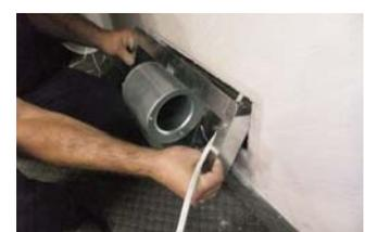
SECURE BLOWER TO WALL AND CONNECT 120 VAC POWER SOURCE TO BLOWER MOTOR LEADS.
