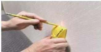
USE STUD FINDER TO DETERMINE CENTER OF STUDS IN CAVITY.
