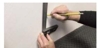
MARK A LEVEL LINE 3 5/8" STRAIGHT ABOVE AND BELOW GRILLE CENTER HOLES. LEVEL TOPS & BOTTOMS OF LINES ACROSS.
