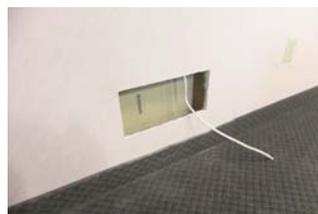
PROVIDE SWITCHED 120 VAC POWER SOURCE LEAD FOR BLOWER.
