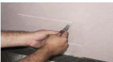
CAREFULLY CUT BLOWER OPENING IN SHEETROCK ALONG HORIZONTAL LINES AND CONNECT ENDS VERTICALLY.
