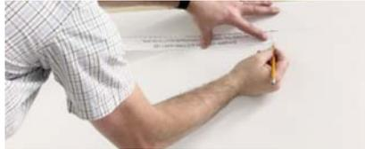
CENTER DIFFUSER TEMPLATE ALONG SHEETROCK CUT AND MARK 4 CORNERS. CUT OUT DIFFUSER OPENING. (1 1/4" HIGH x 13 5/8" WIDE)
