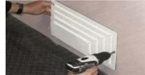
ATTACH GRILLE TO WALL WITH PROVIDED SCREWS.
