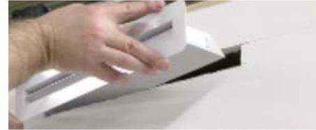
INSERT DIFFUSER INTO WALL WITH AIR SCOOP POINTING TOWARDS BLOWER.
