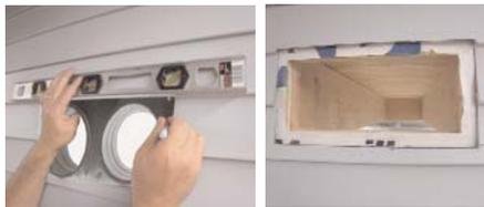
LEVEL XCHANGER HOOD BACKING PLATE AND TRACE FLANGE. TRIM SIDING BACK SO BACKING PLATE CAN BE MOUNTED FLUSH TO EXTERIOR SHEATHING.
