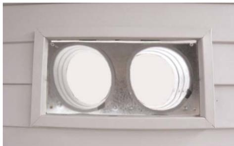
INSTALL J CHANNEL OR APPROPRIATE FLASHING AROUND XCHANGER HOOD BACKING PLATE.
