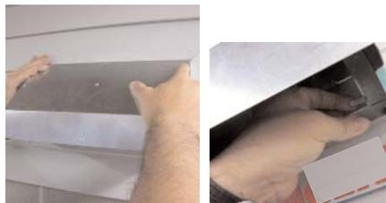
HOOK X2R HOOD ON BACKING PLATE TOP FLANGE. INSTALL (4) KEPS NUTS ON BACKING PLATE STUDS AND TIGHTEN HOOD TO BACKING PLATE.
