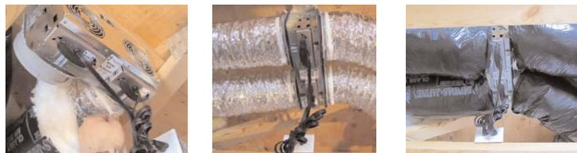
FIRMLY SECURE DUCT TO COLLARS WITH INCLUDED ZIP TIES. INSULATED FLEX SHOULD BE USED IN COLD CLIMATES TO PREVENT CONDENSATION. PROPERLY SUPPORT DUCT TO MINIMIZE SAGGING, BENDS AND SHARP TURNS THAT MAY RESTRICT AIR FLOW.
