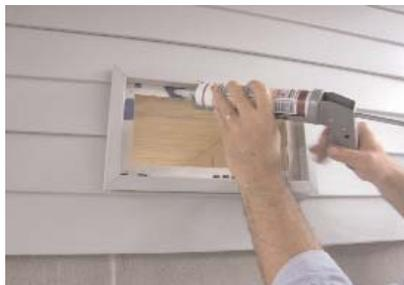
PLACE A BEAD OF CAULK ON XCHANGER HOOD BACKING PLATE FLANGE OR BUILDING SHEATHING BEFORE INSERTING BACKING PLATE.
