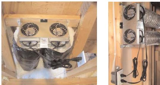
MOUNT X2R BELOW OR BETWEEN JOISTS / TRUSSES TO A CROSS BRACE OR ON A STUD WALL IN ANY ORIENTATION. USE (3) 5/16" X 1 1/4" SCREWS ON LEFT, RIGHT AND CENTER MOUNTING FEET.
