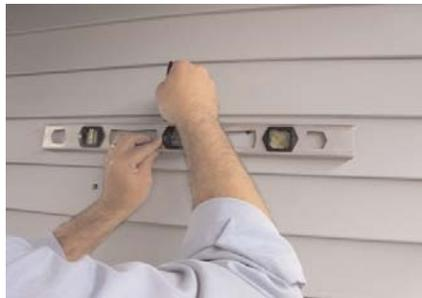
DRILL (4) 1/2" CORNER HOLES THROUGH WALL FROM INTERIOR AND CONNECT HOLES ON EXTERIOR WITH A LEVEL. ALIGN TEMPLATE WITH HOLES AND TRACE REMAINING LINES.
