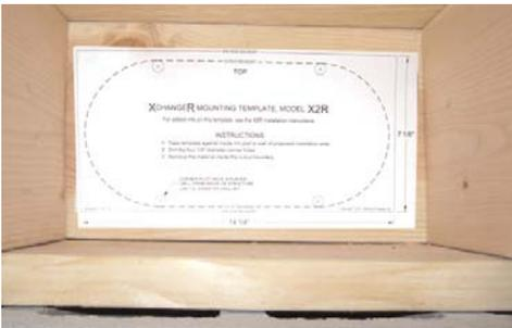
CENTER AND LEVEL TEMPLATE BETWEEN JOISTS / TRUSSES OR PLACE ON WALL X2R XCHANGER WILL EXIT.
