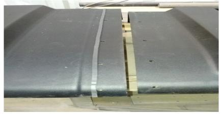
3. Place roof sections together and secure one to the other with  $\frac{1}{2}$ "-20x  $\frac{3}{4}$ " long bolts through the top side with a  $\frac{1}{4}$ " SAE flat washer on top and bottom and the  $\frac{1}{4}$ "-20 acorn nut on the bottom side of the roof. This works best starting from the middle outwards. (Leave out the 3 and 4 bolts from the front. These holes are for a mounting bracket.)
