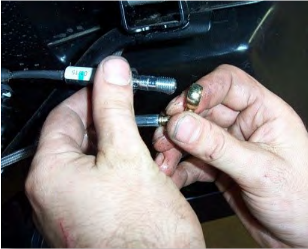
Install the new longer 48" brake line (45X) on the right side of the UTV.
