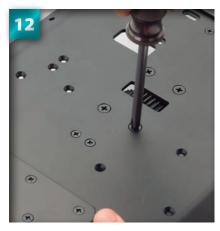
Screw the remaining 4 x 16mm self-tapping countersunk screws into the remaining three holes. When all are in, tighten each fully.
