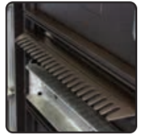
Aluminum comb prevents mail fishing from the outgoing mail collection compartment.
