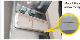
Mount the sensor horizontally with the arrow facing DOWN, as shown.
