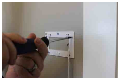
Secure wall mount to the wall with provided hardware
